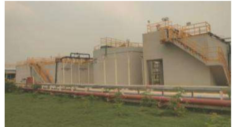
Advanced Waste Water Treatment Plant (RO & MBR) (Recycling ratio - 65%)
